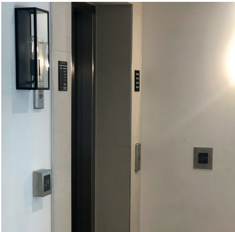
Lift calling is also proximity reader controlled.
