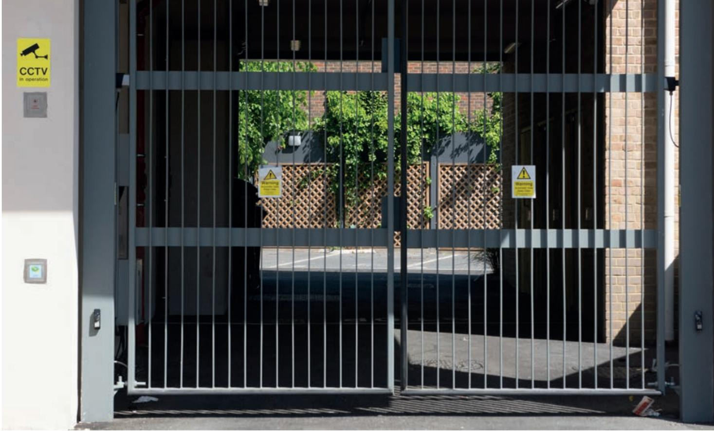
Right leaf of vehicle gate opens when proximity reader is used by cyclists, both leaves open when radio transmitter is used by motorists. All controlled by the IPGUARD® smart system and remotely programmable!
